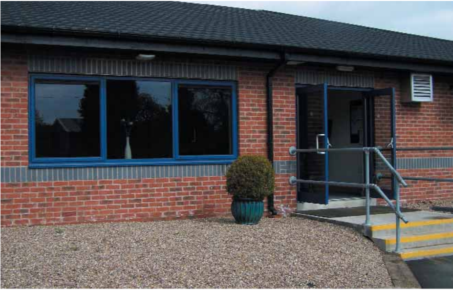
SOUTHWELL New stable staff canteen.
